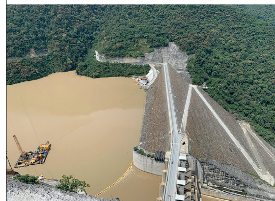
Fig. 3. The Ituango water intakes in relation to the other structures.
