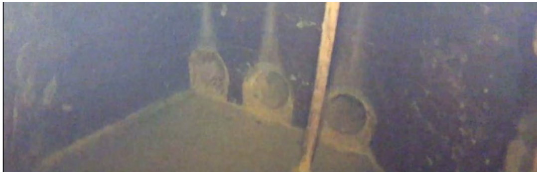
Figure 3-3: Pipes in west outlet from upstream
