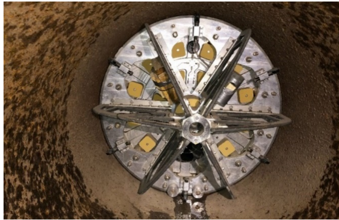
Figure 2-3: Installed 72-inch (1.8 m) isolation barrier, from downstream
