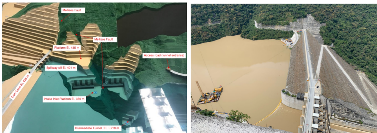
Figure 5-1: The water intakes in relation to other structures
