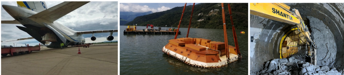
Figure 5-4: Transport in cargo plane – Immersion – Demolition of the concrete plugs
