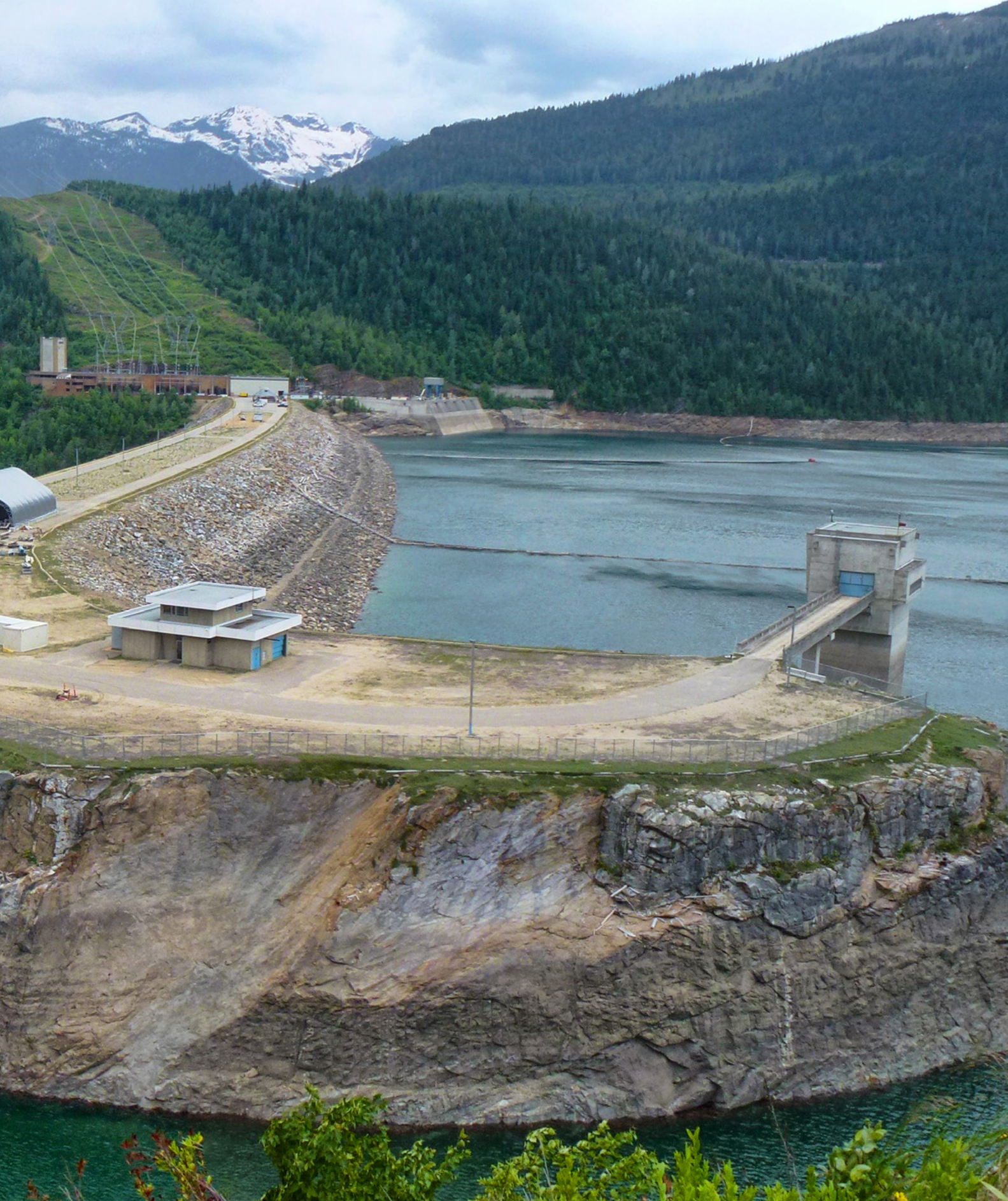
MICA DAM, BC, CANADA - 1,736 MW
