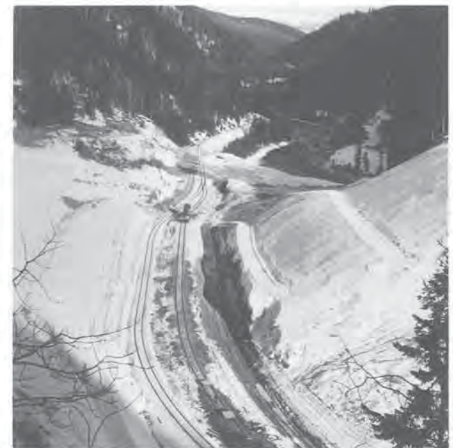
CN Rail, Messiter Tunnel removal, Blue River, B.C., 1963 Photos: Mark Olsen
