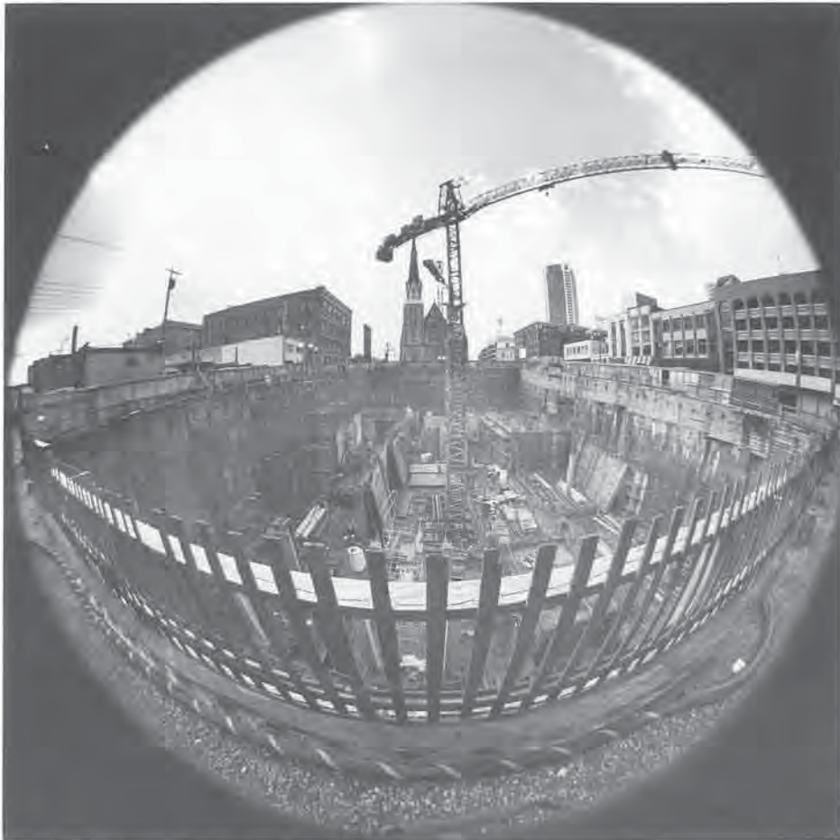
Cathedral Square substation, Vancouver, B.C. – Twenty-metre-deep excavation and shoring, February 17, 1982.
