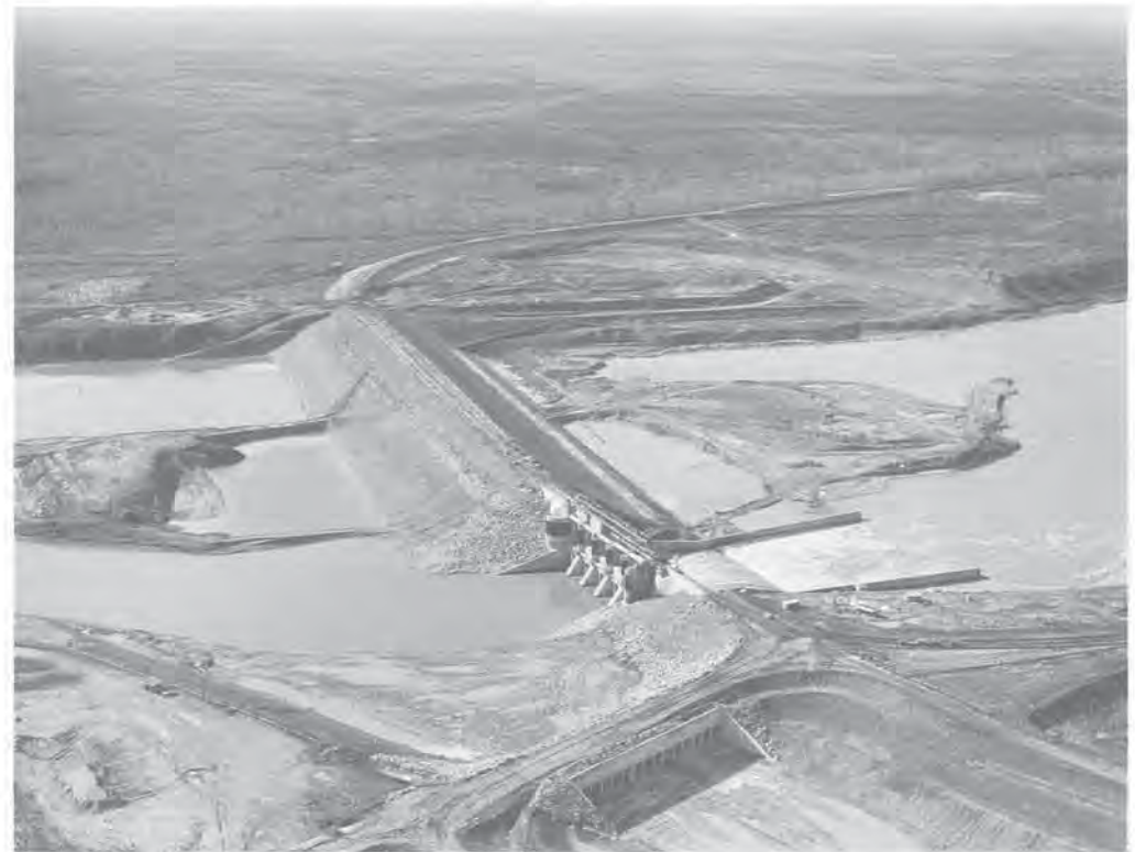
Under construction, October 25, 1962.
