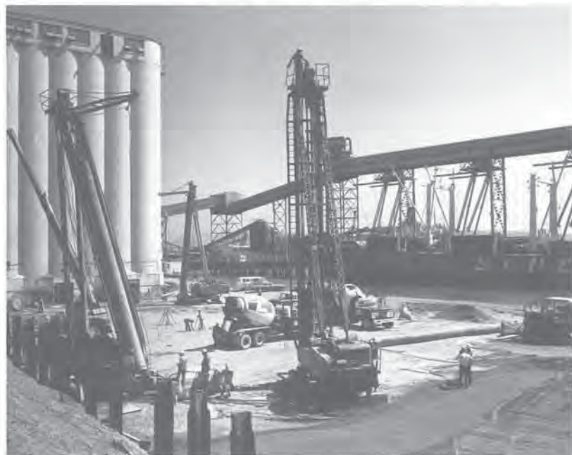
Driving Franki piles, Saskatchewan Wheat Pool extension, North Vancouver, B.C., 1977.
