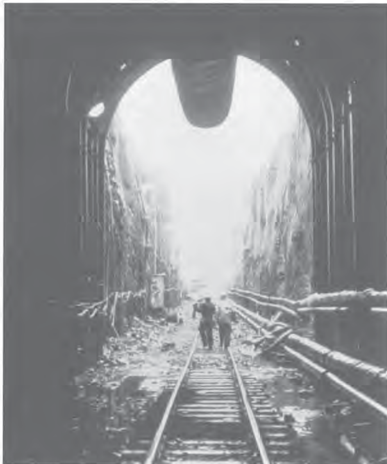
B.C. Rail Tumbler Ridge Branch Line, Wolverine East Tunnel, 1983. Photo: Raymond Benson.
