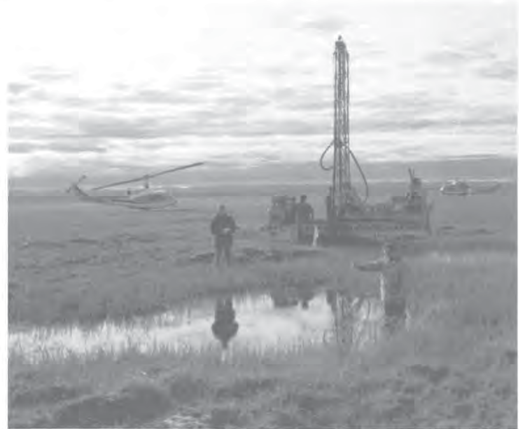
Mackenzie Valley Oil Pipe Line terrain evaluation: Soil sampling on North Slope of Alaska using heli-drill, August 1970. Photo: Donald Davison
