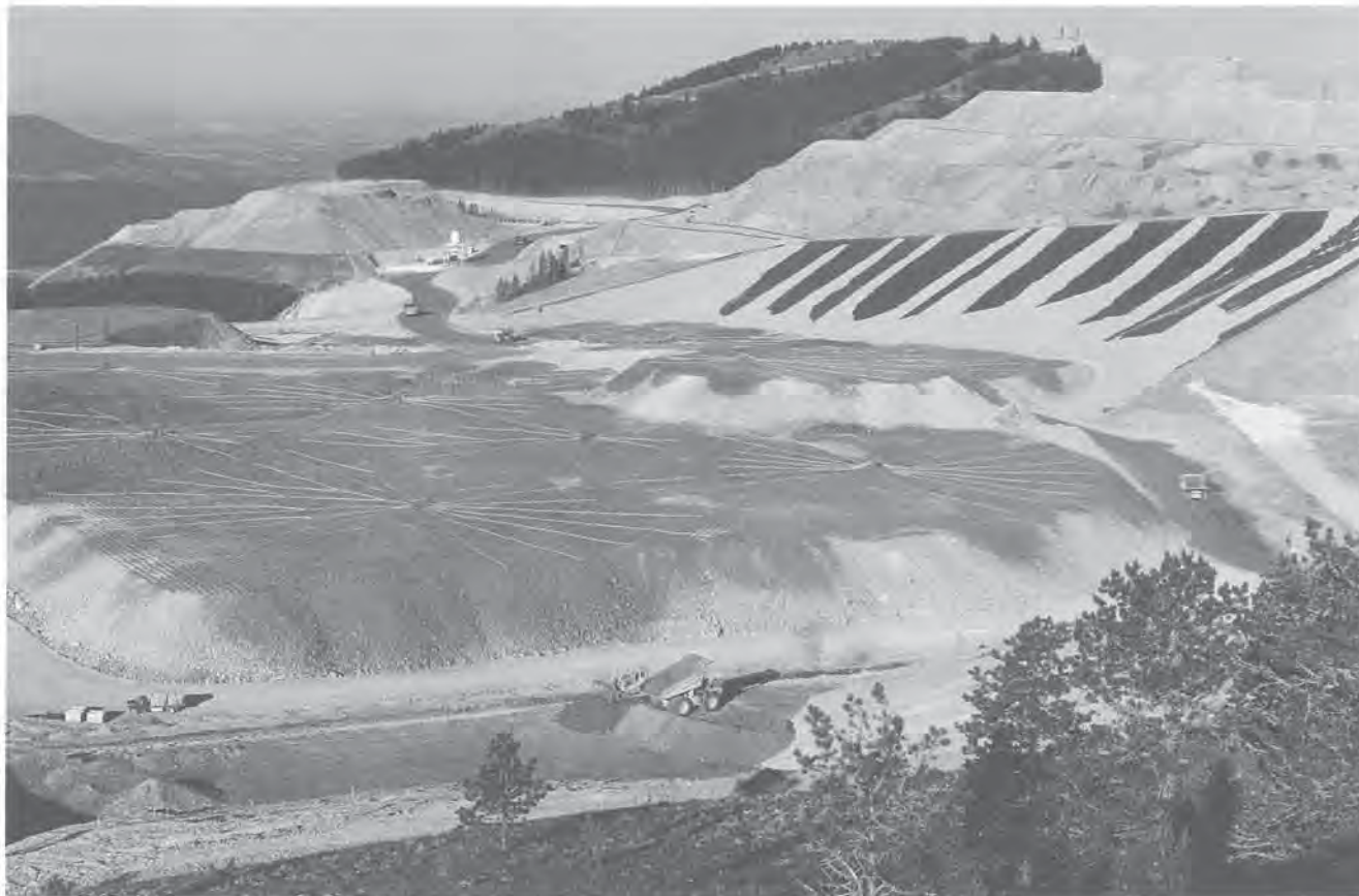
Landusky heap-leach, stage II construction, Little Rocky Mountains, Montana, July 12, 1991.
