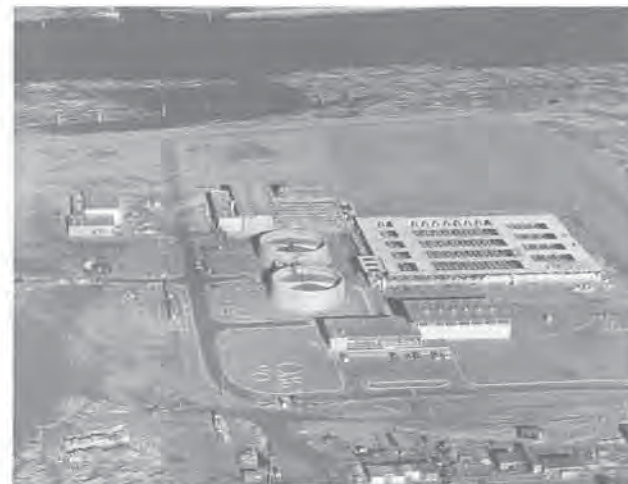
Plant construction nearing completion, January 28, 1963.
