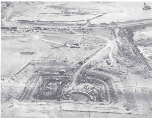
Excavation for deep pumphouse, August 21, 1961.
