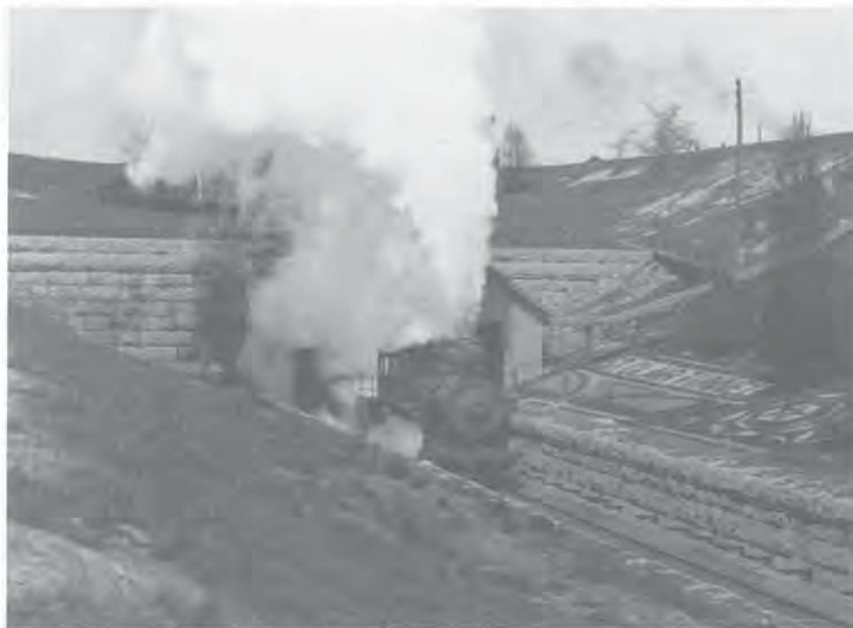
St. Clair Tunnel Company 0-10-0 engine emerges from the Sarnia Portal “amid a cloud of steam and smoke,” ca. 1900.
