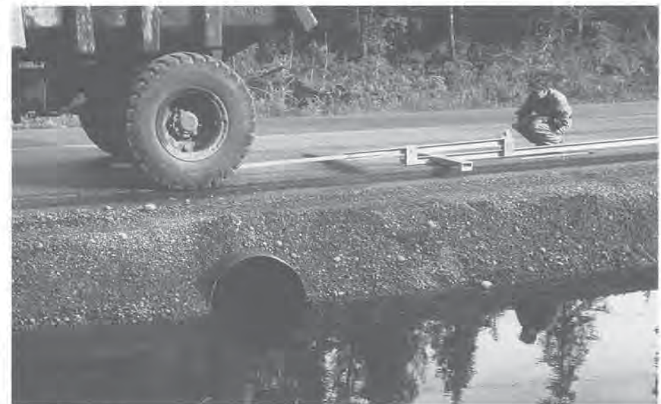
Cyril Leonoff measuring pavement deflection with Benkelman beam, Kitimat, B.C., fall 1953.
