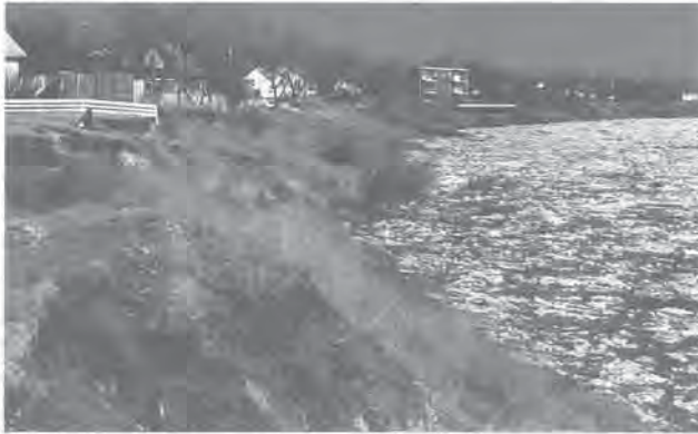
Eroded bank before stabilization, April 1976.
