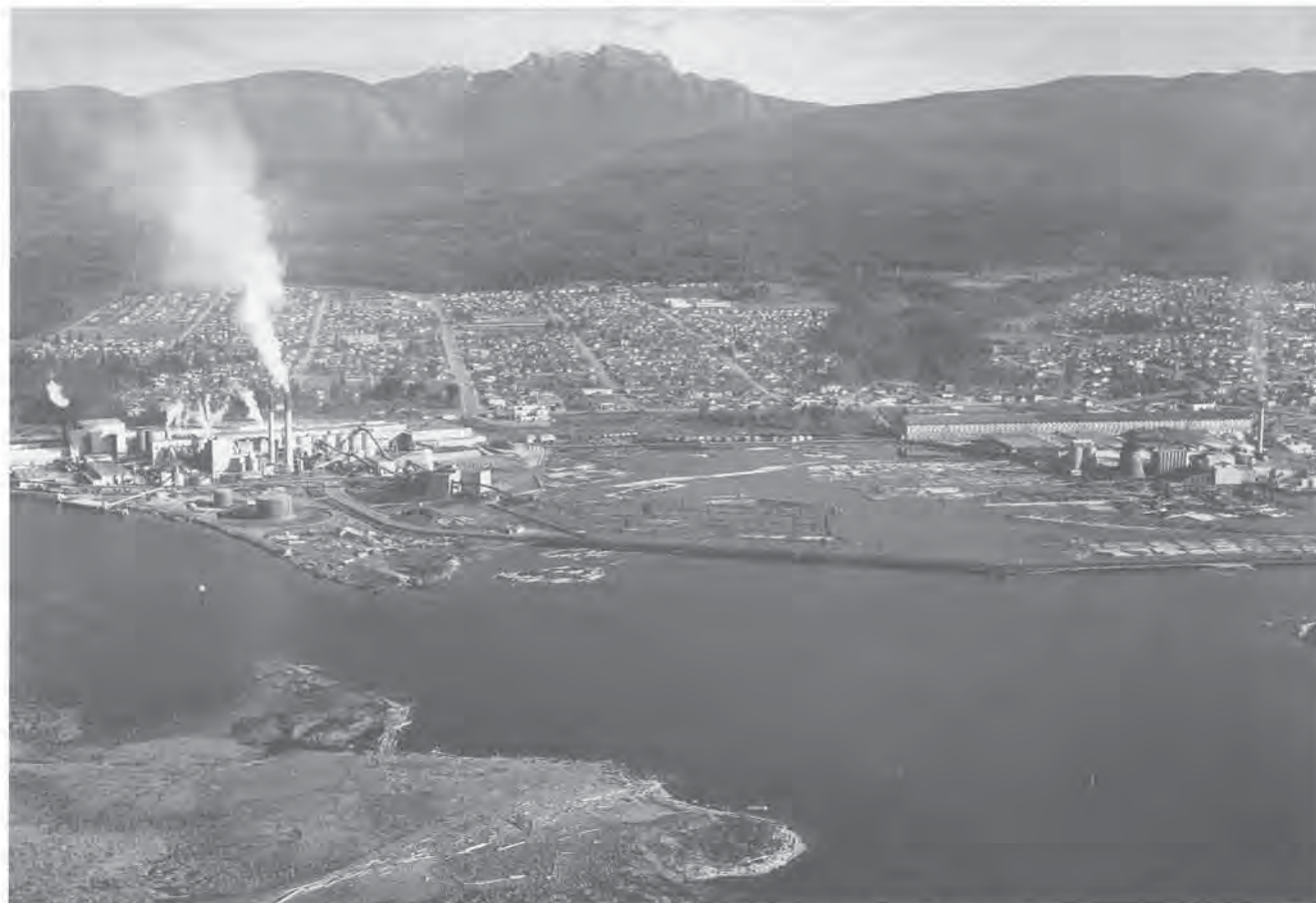
Macmillan, Bloedel and Powell River Ltd., pulp and paper mill, Port Alberni, B.C. – Mill buildings, foreshore fill, and deep-sea dock trestle, November 4, 1959.
