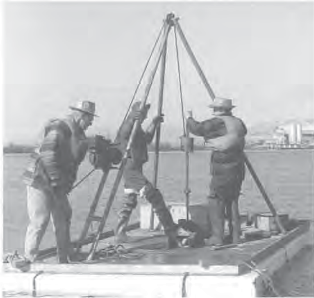
Light drill rig – On Styrofoam raft, piston sampling for borrow material in the Fraser River, March 1960.
