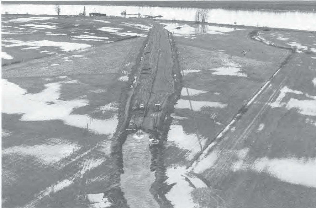
Hydraulic fill placement of roadbed, January 16, 1961.
