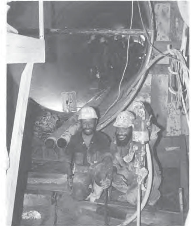
Ok Menga project, native workers at lower end of steel penstock at powerhouse, February 1, 1988.
