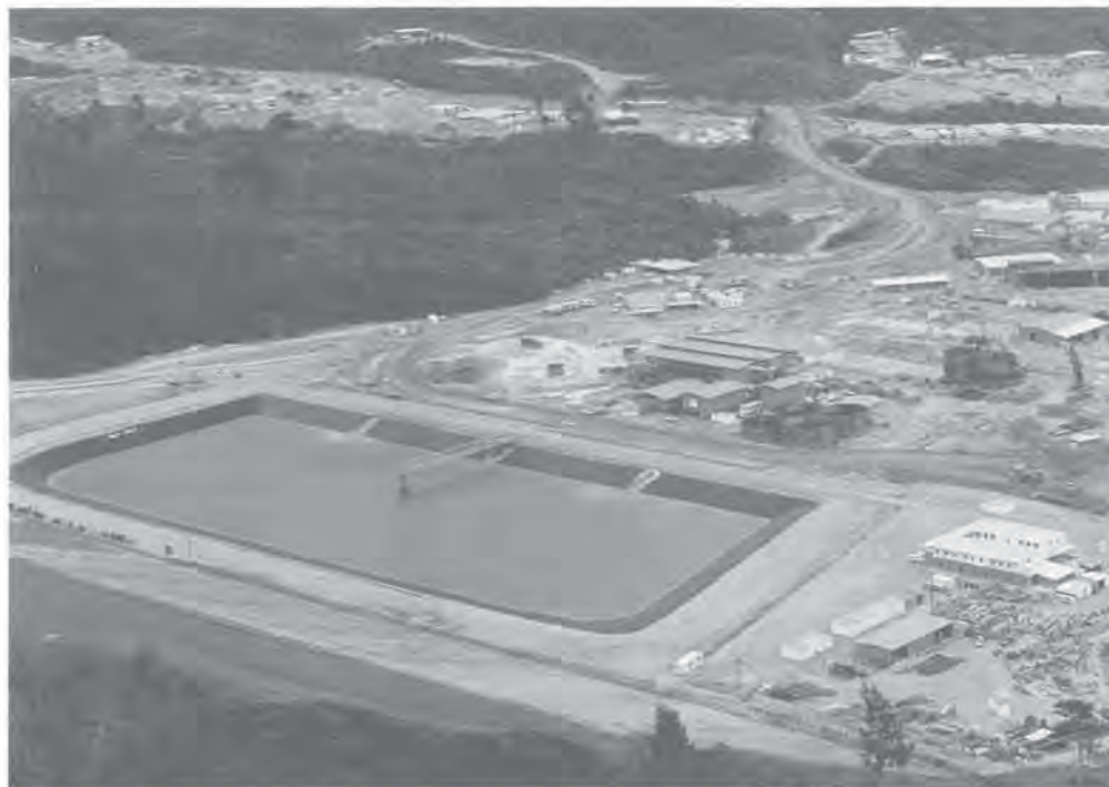
Porgera Gold Mine containment pond for gold ore slurry, Papua New Guinea, 1990. Photo: Placer Dome Inc.
