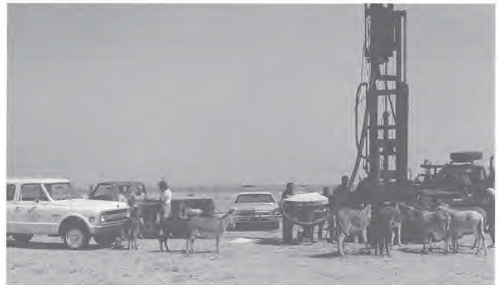
Construction materials inventory, State of Kuwait – Drilling in desert using Becker hammer drill with cyclone, Bedouin camp in background, 1974.
