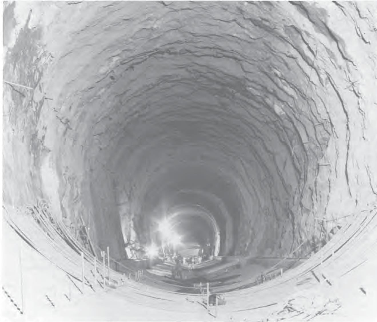
Betania hydroelectric power tunnel, Colombia, September 1983. Photo: Sedic
