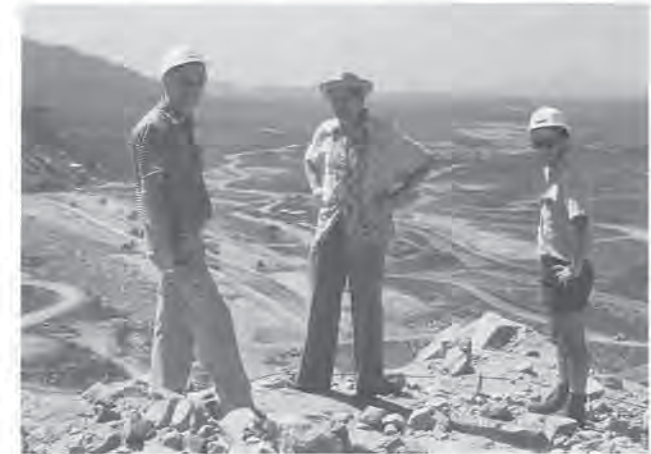
Inspecting site construction, from left: Louis LaFlamme (Concept Canada), Cyril Leonoff, Gordon Gullan (resident engineer), March 2, 1982.
