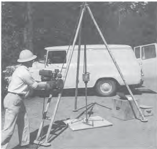
Light drill rig – Driving cone penetrometer.
