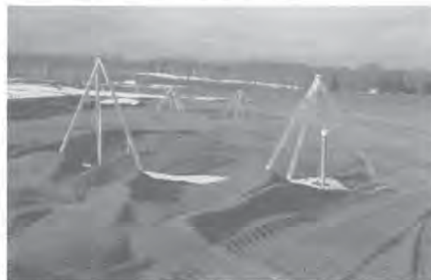
Settlement plates and standpipe piezometers.
