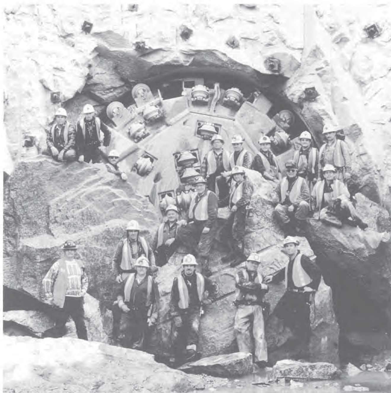
Breakthrough by Tunnel Boring Machine (TBM) of Kemano power tunnel, June 25, 1991.
