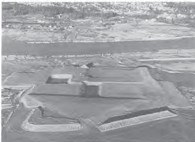
Preload fill in place, December 3, 1960.
