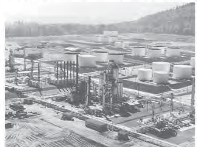
British-American Refinery, Port Moody, B.C., 1958.
