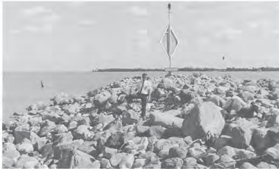
Winnipeg Beach, Manitoba breakwater, July 1969. Photo: Cyril Leonoff
