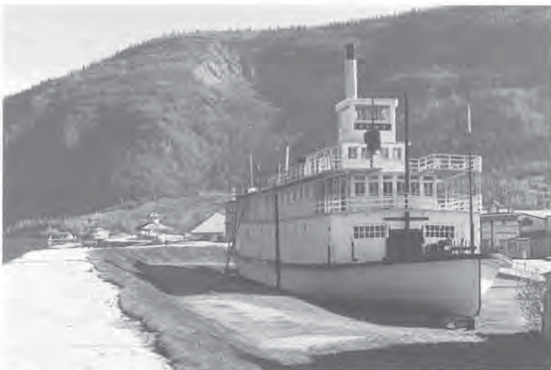
The aesthetically pleasing dyke protects the S.S. Keno National Historic Site, July 1988. The Keno was the last sternwheeler to ply the Yukon River, from Whitehorse to Dawson City on August 29, 1960.
