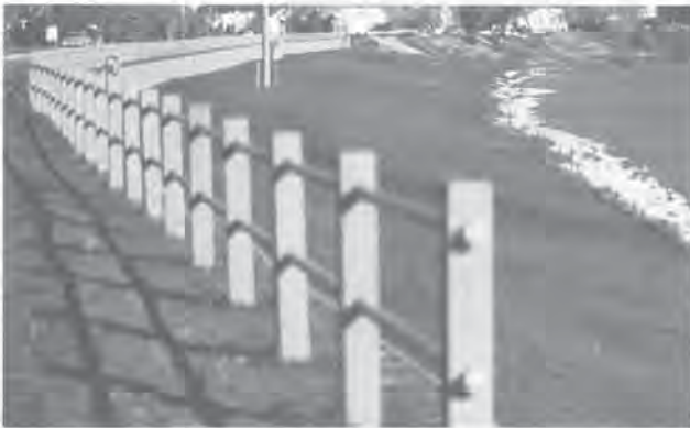
After remediation, October 1977.
