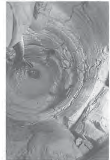
Rock-socketed caisson installation, University of Winnipeg, 1970.
