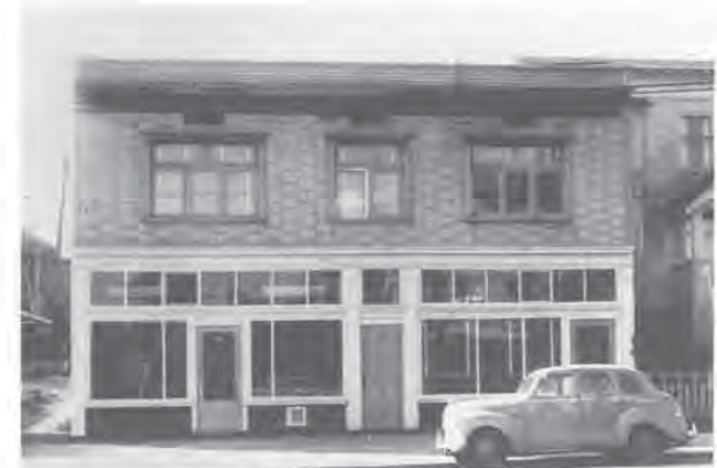
Ripley and Associates offices at 1930 West Broadway, Vancouver, B.C., shortly after occupation, 1953. Klohn’s A-40 Austin in front.
