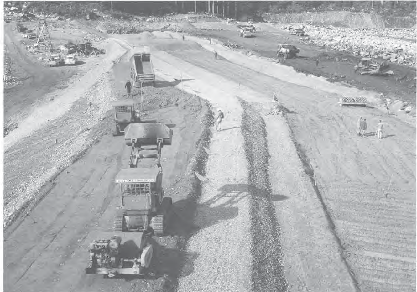
Zoned construction, Seymour Falls Dam, Greater Vancouver Water District.
