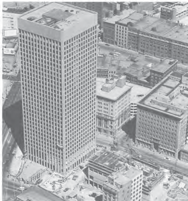
Richardson Tower, construction nearing completion. Photo: Ralf Lilje-Gren
