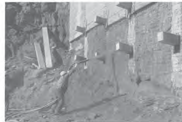
Cathedral Square substation, Vancouver, B.C. – Shotcrete application.
