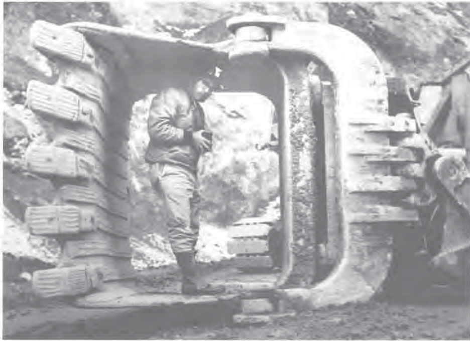
Mark Olsen demonstrating size of shovel bucket, Mission Dam, November 19, 1957.
