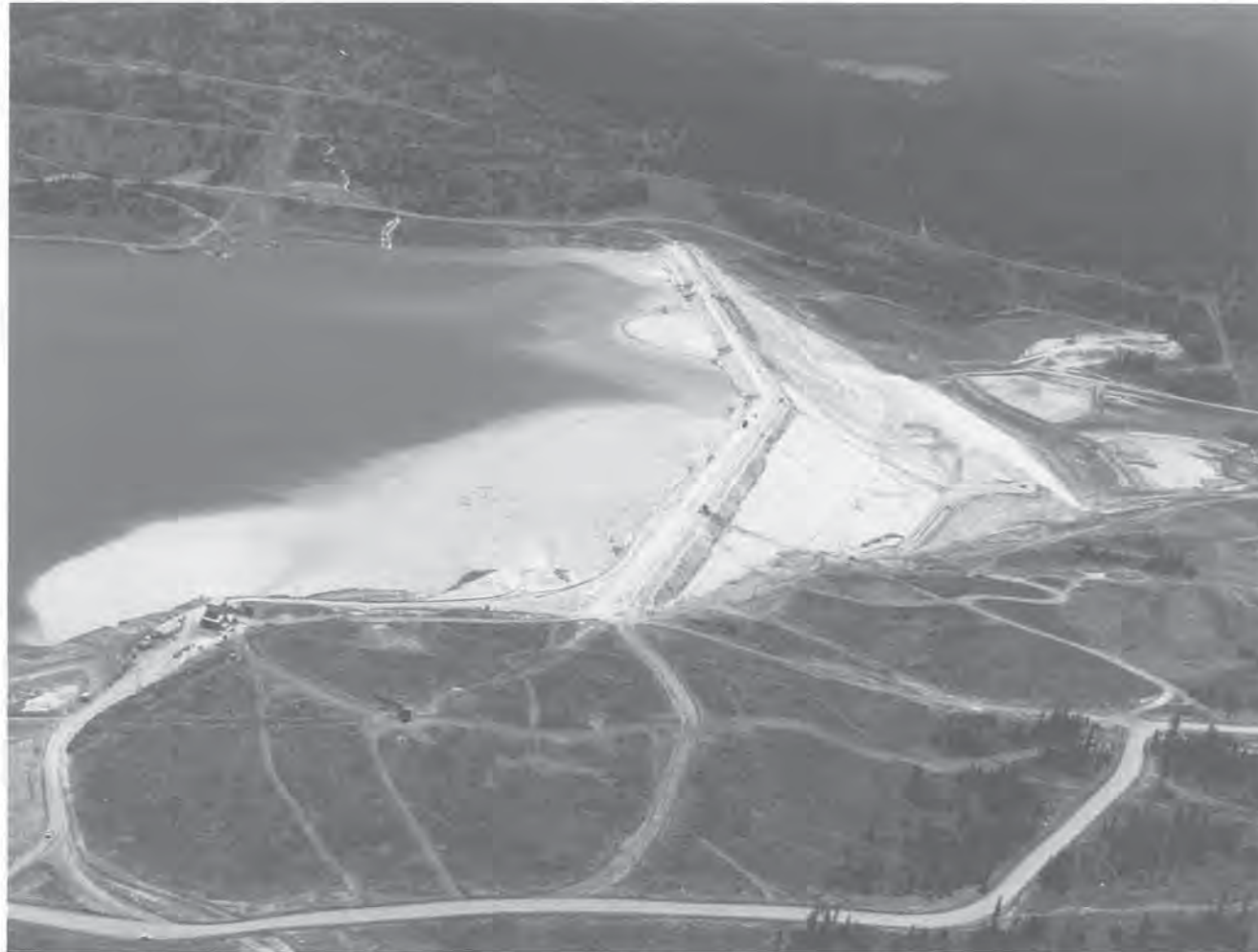
Valley Copper L-L Dam, Highland Valley, B.C., 1988. Photo: Valley Copper
