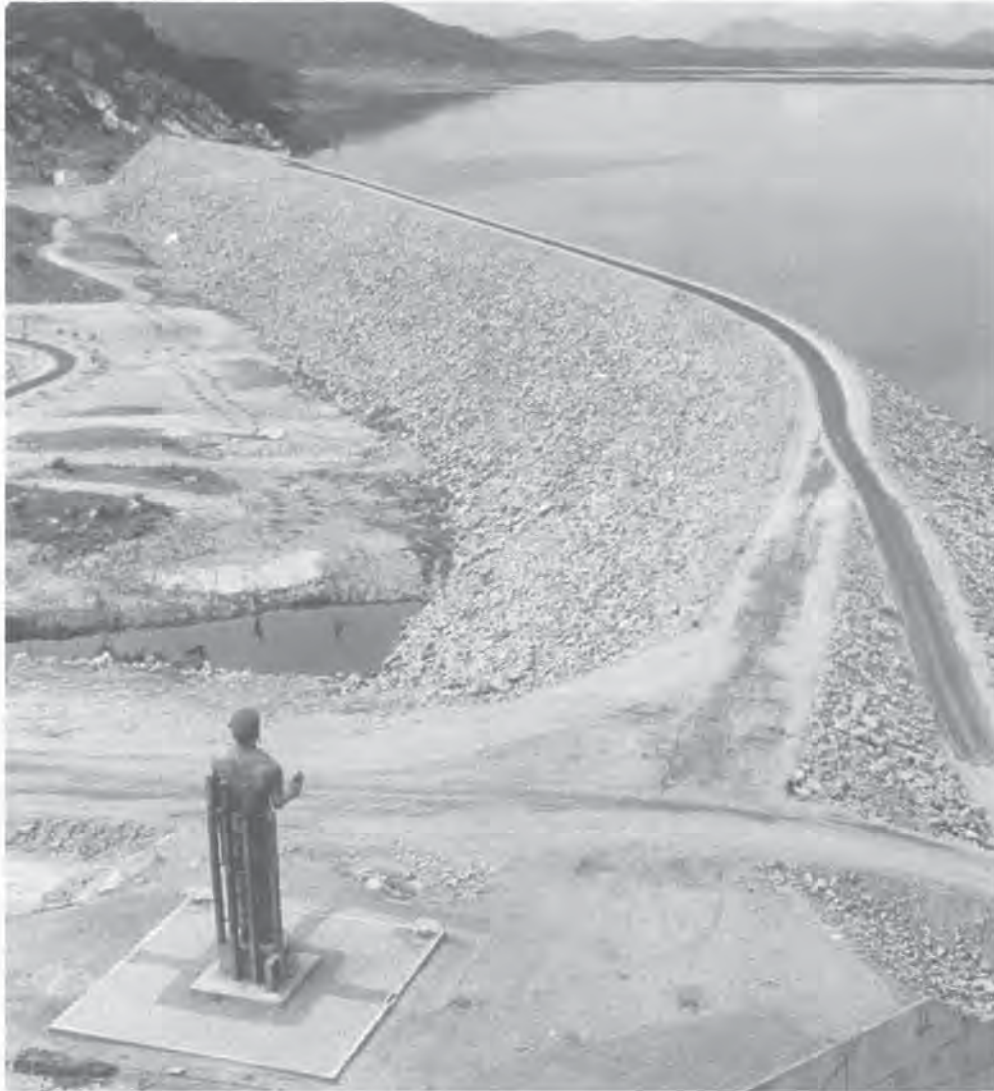
Maduru Oya reservoir project, Sri Lanka – Rockfill dam on completion, 1983.
