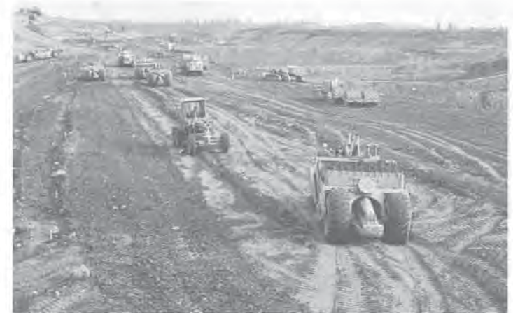
Placement of compacted earthfill.
