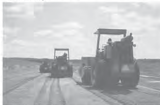
Vibroller compaction of starter-dam fill.
