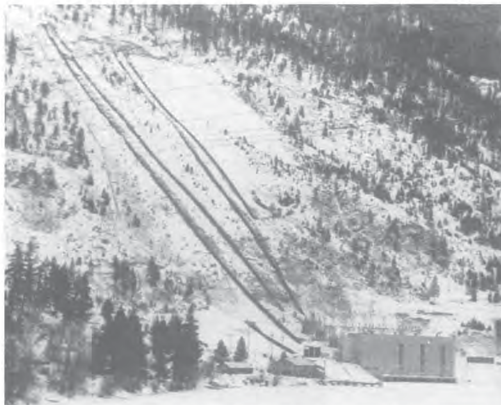
Powerhouse and penstocks, Bridge River development, Shalalth, B.C., February 22, 1956.
