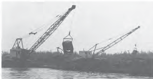
Double-casting of excavated peat by two draglines.
