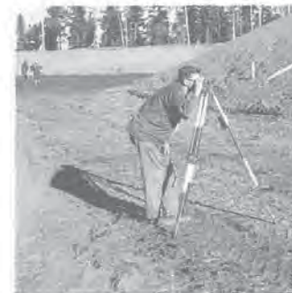
Donald Davison running levels on top of impervious lining, September 14, 1956.
